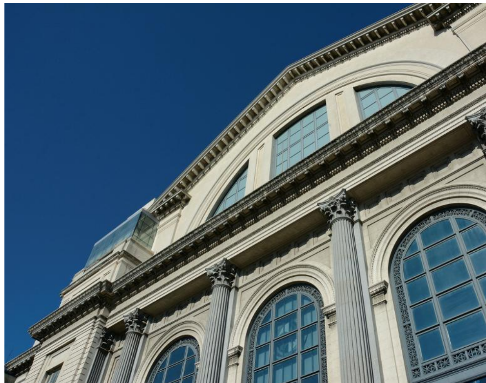
Counter facade of BROU Head Office
